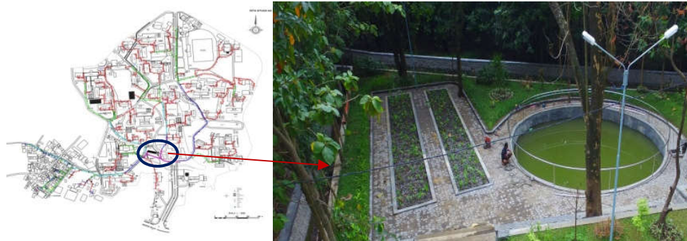
Figure 4.A. Integrated Liquid Domestic Waste Treatment, which manages liquid domestic waste from campus and surrounding areas in Jebres District (sources: Ministry of Public Works and Spatial Planning, 2017)
