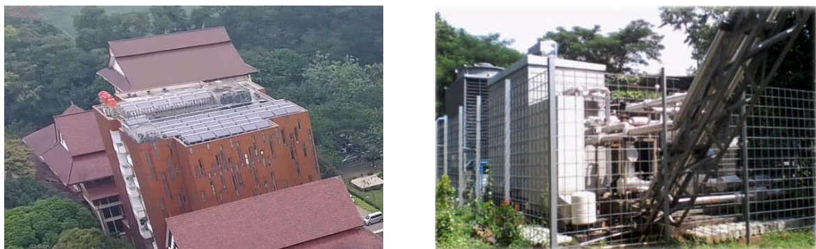
Figure 6. Solar cooling absorption chiller system at the Manufacturing Research Center (MRC) building, Faculty of Engineering, Universitas Indonesia
