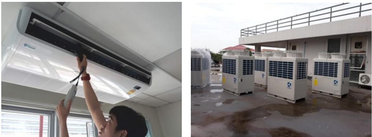
Figure 4. Air flow rate measurement and VRF condensing unit installation
