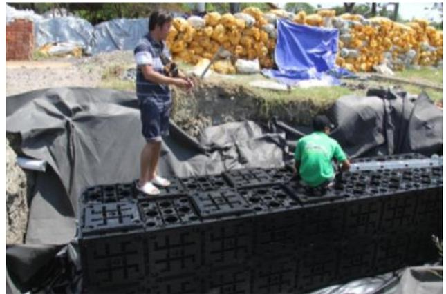
**Fig. 4.** Urban farming ITS products and underground tanks to harvest rainwater
