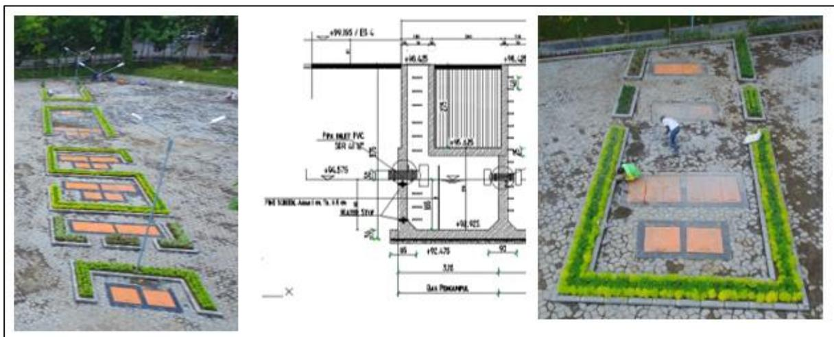
**Fig.4 .** Unit of anaerobic domestic liquid waste water treatment UNS.
