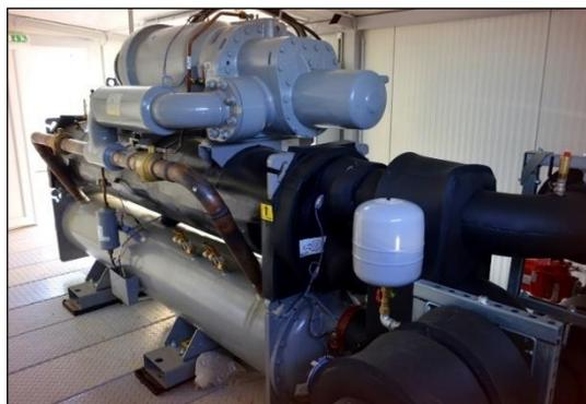
**Fig. 3.** Heat pump for usage of wastewater heat
