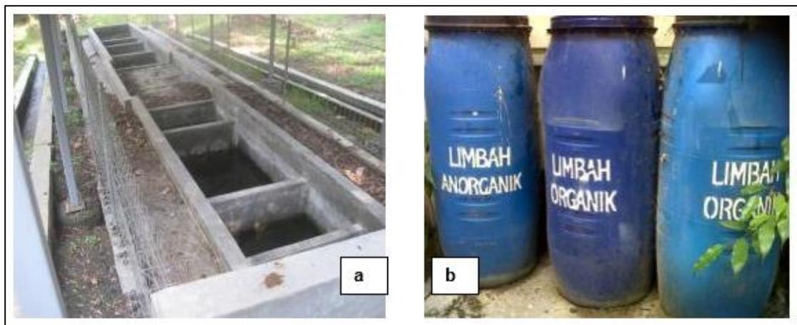
**Fig.5** . (a) Toxic waste treatment pond for decomposition process in the Center of Laboratory in MIPA Faculty. (b) toxic waste treatment by collecting waste into tank
